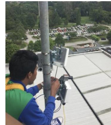
Figure 03 | Installation of Terragraph nodes
